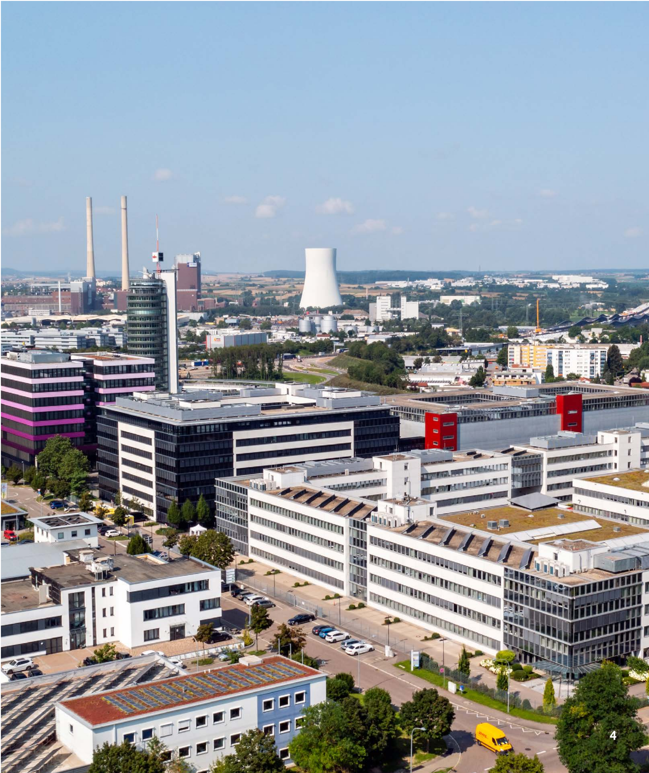
The Lidl Stiftung & Co. KG administration building in Neckarsulm is the heart of sustainability management for the companies of Lidl Group.
